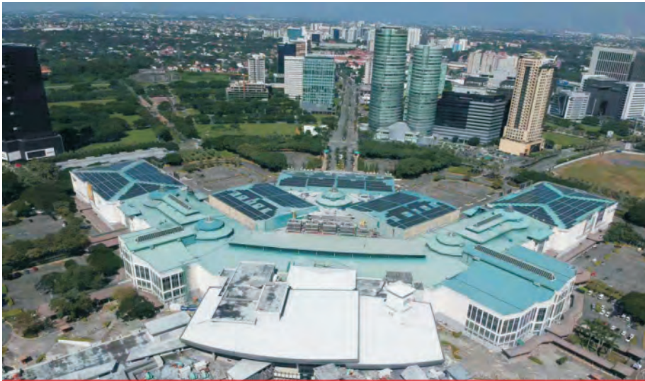
CASE STUDY: Festival Supermall Alabang Solar Rooftop, 2.8MW
